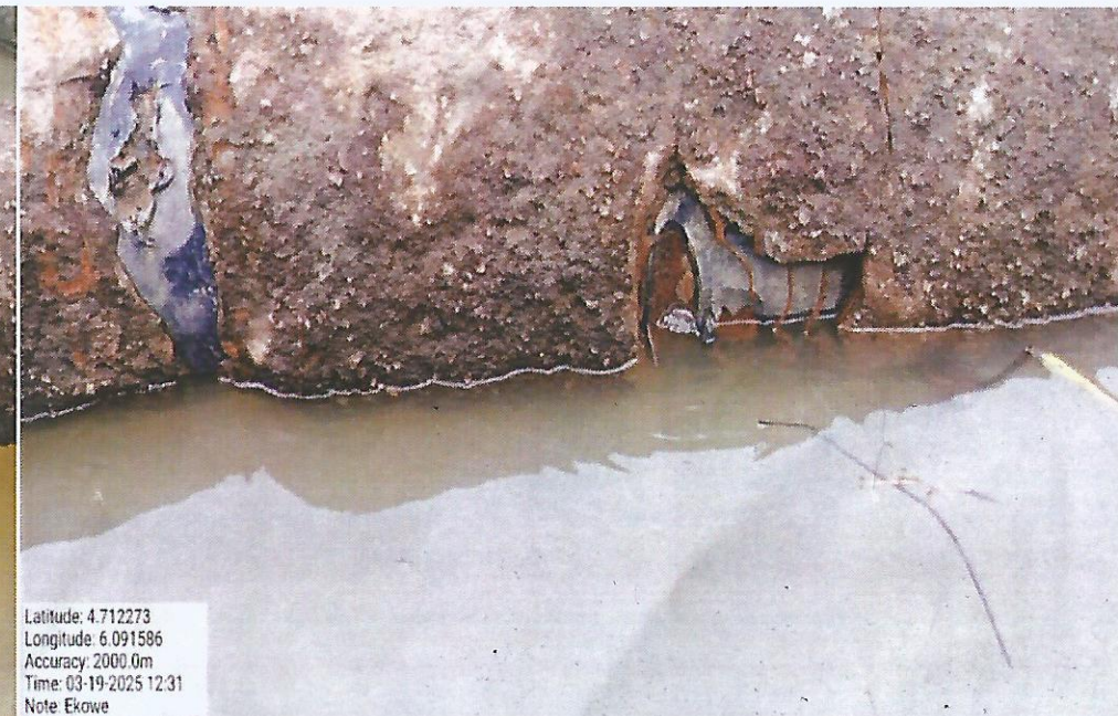
EXPOSURE OF THE INCIDENT POINT 10" DIEBU CREEK - NUN RIVER DELIVERY LINE RIGHT OF WAY AT EKOWE RIVER CROSSING
